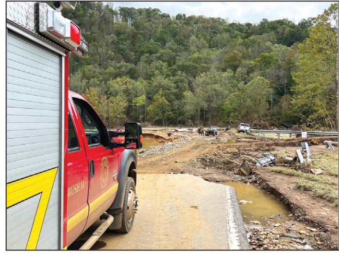
Hwy 19W Bridge at Langford Branch Road
