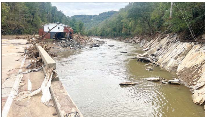
Hwy 19W Bridge Gone at Soup House
