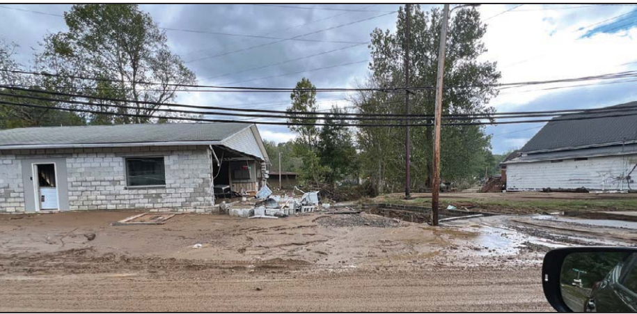
Where the Micaville Post Office was located, building completely gone
