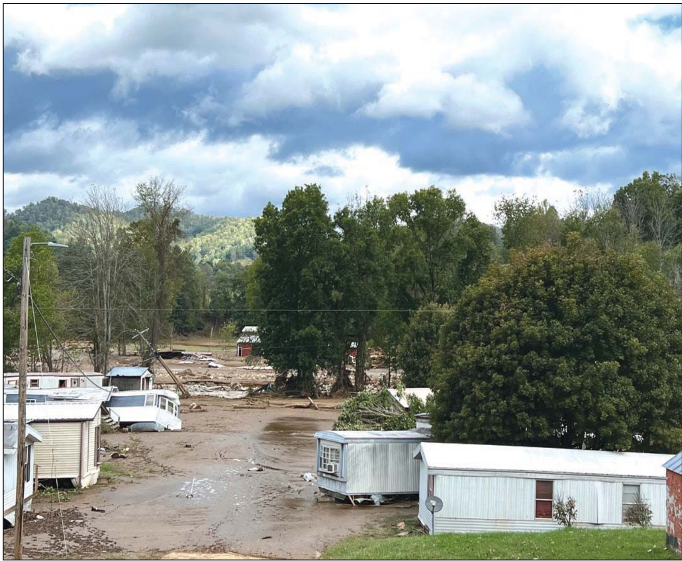
Riverside Trailor Park
