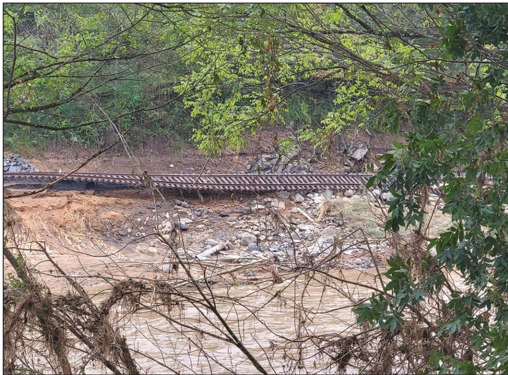
Railroad tracks are damaged, the state bridge crossing the river at OC Whitson Store is gone.
