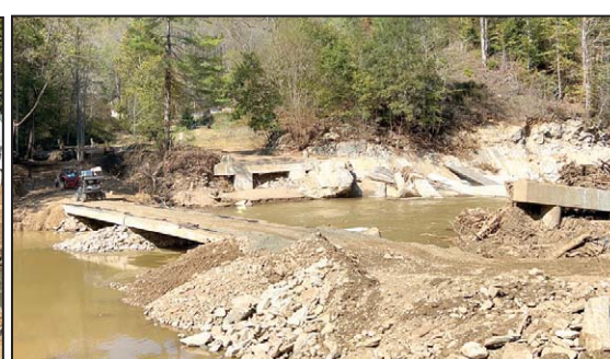
The group came across this low water bridge which had just been completed the night before, allowing these residents their first roadway access out since Helene hit on Sept. 27th.
