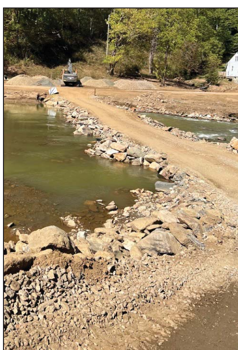
Low water access across a section of the Cane River has been built.
